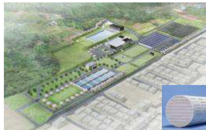
▲ Aizuwakamatsu City: Renewal project of Takizawa Water Purification Plant
