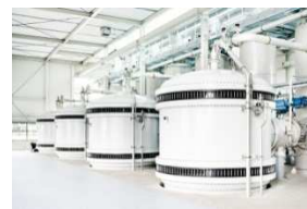
▶ CeraMac® and Ceramic membrane (Delivered to water treatment plants in Andijk, the Netherlands)
