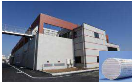
▲ Yokohama City: Redevelopment project of Kawai Water Purification Plant
